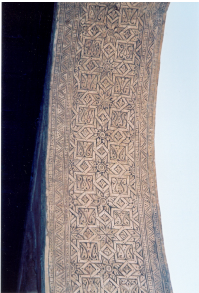
Figure 49: Detail of the plaster reliefs found on the many arches of the arcades
