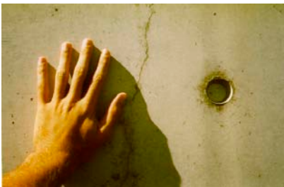
Figure 3: Detail of my hand's relationship with the concrete of Tadao Ando's Conference Centre, Vitra Design Museum, Basel
