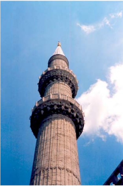
Figure 19: Detail of one of the six minarets
