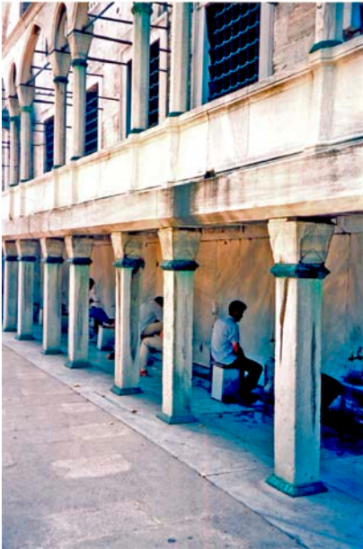
Figure 17: The washing spigots being used on the exterior of the Mosque
